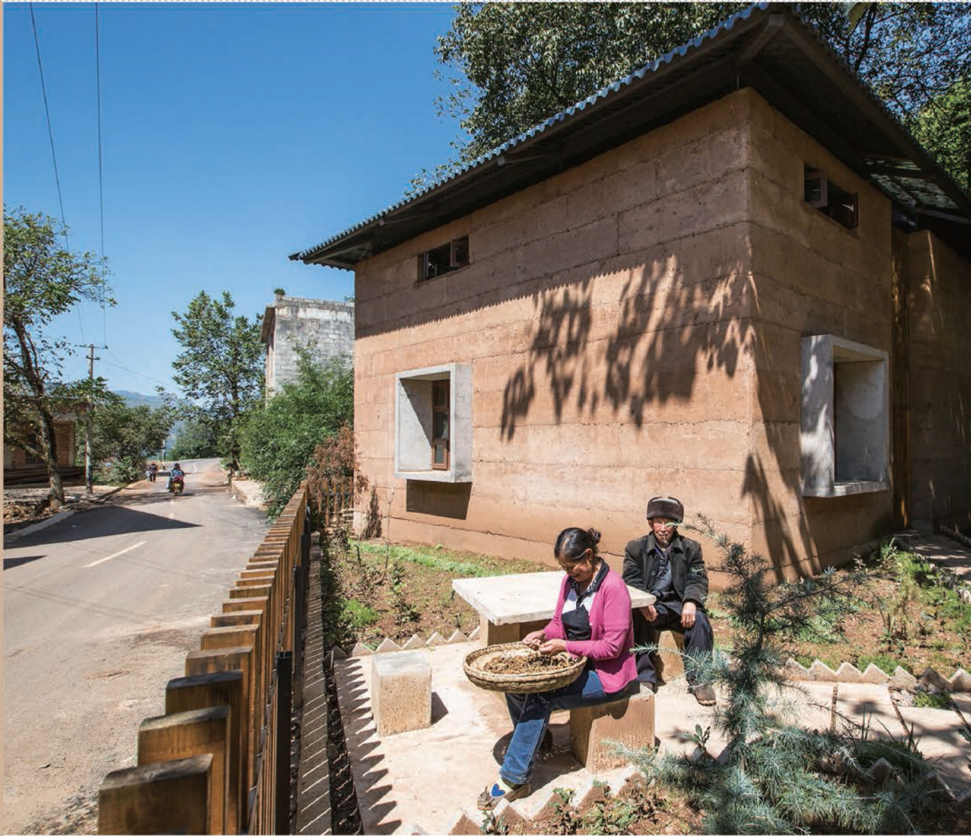
Figure 4: Entrance and courtyard of prototype house
